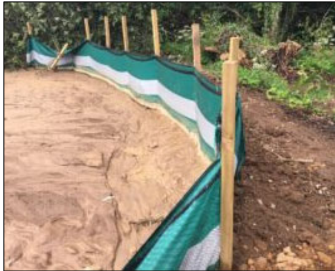
Figure 2-3 Typical Silt Fence
