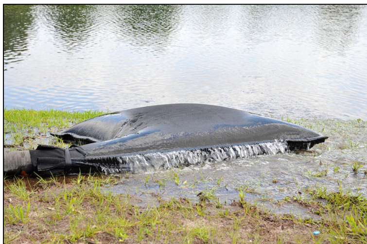
Figure 2-2 Typical Silt Bag
